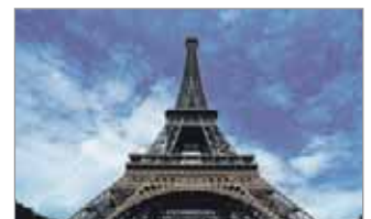
For safely going up and down: KABELSCHLEPP in the Eiffel Tower, Paris.
