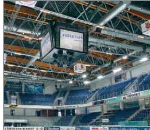
UNIFLEX cable carrier system in a zig-zag system on a lowerable multimedia cube in the Nuremberg Arena
