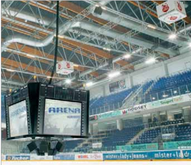
UNIFLEX cable carrier system in a zig-zag system on a lowerable multimedia cube in the Nuremberg Arena
